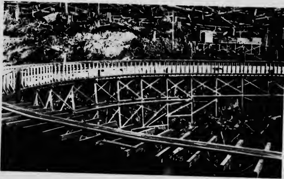
Vancouver Island Power Company Limited. Flume between Jordan River Dam and Forebay Reservoir.
